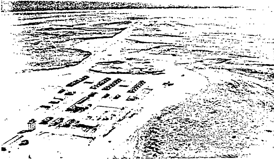
FIGURE 1-44. CONSTRUCTION CAMP ON LIDILBUT (GENE) ISLAND.
