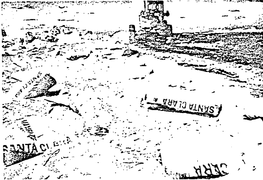
FIGURE 8-30. CEMENT BAGS PLACED FOR SOIL-CEMENT MIX.
