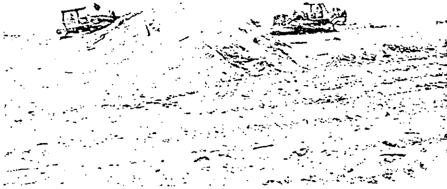
FIGURE 6-7. SOIL WINDROWING.
